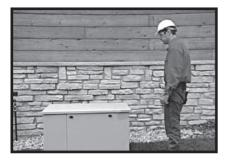
Shut OFF utility power and make sure the generator starts automatically.
